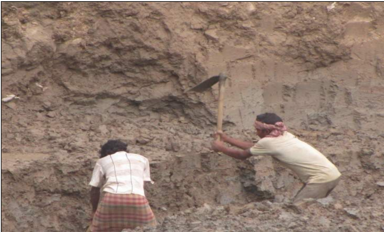
Plate 4. excavation from the natural levee (embankment).
