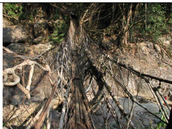
Fig. 3. Preparing root bridge on rusted cable bridges.
