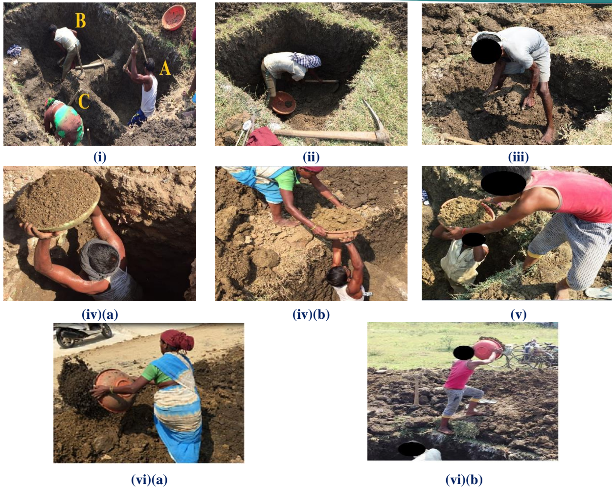
Figure 2. Actual images of performing excavation and associated work
