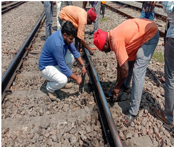
c) Placing rubber pads with gang men.
