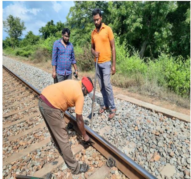
b) Inserting the absorption pads along with gang men.
