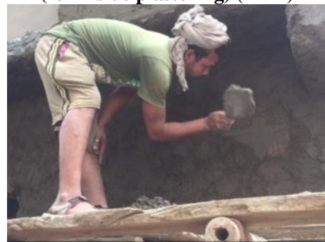
(f) applying mortar on the wall (for outside Plastering) (PL-6)
