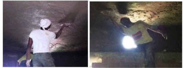
(i) (ii) (b) Level /Plan the mortar (PL-2)
