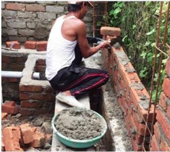
c) Filling bricks gap (BL-3)
