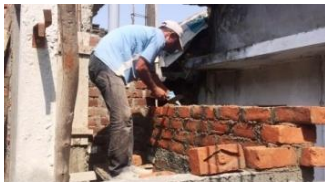
(b) laying of mortar bed (BL-2)
