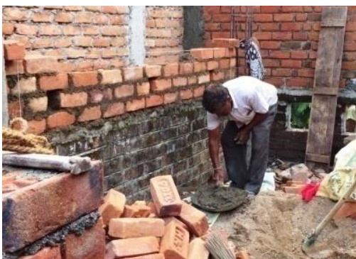
(a) Collect mortar from iron pan (BL-1)
