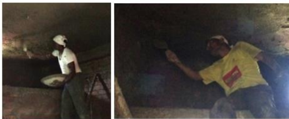
(i) (ii) (a) Applying mortar to ceiling (PL-1)
