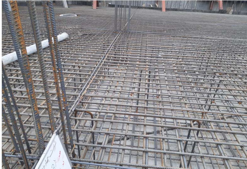
Fig. 3. Rebars used for implementing CEGE
