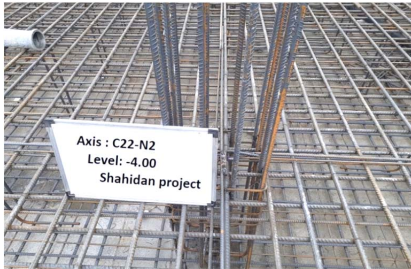
Fig. 2. Rebars used for implementing CEGE
