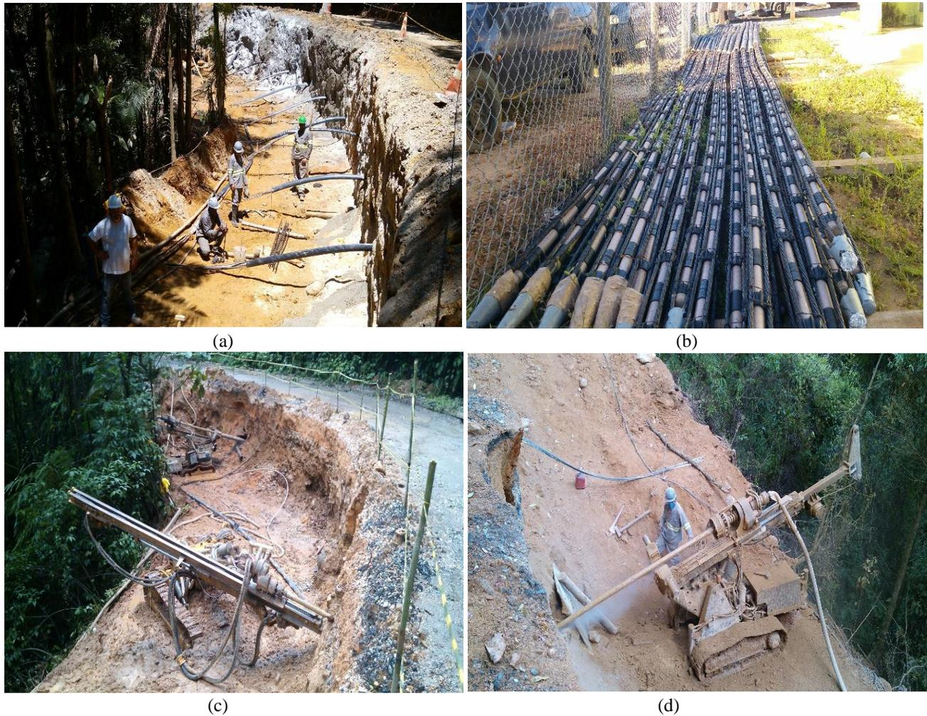
Figure 4. (a) Tie line, (b) overview detail of tie line, (c) detail of machine supported on berm, (d) drilling with compressed air.
