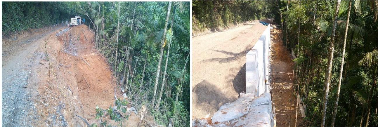
Figure 2. (a) General view of slippage, (b) General view of hillside recovery with curtains.
