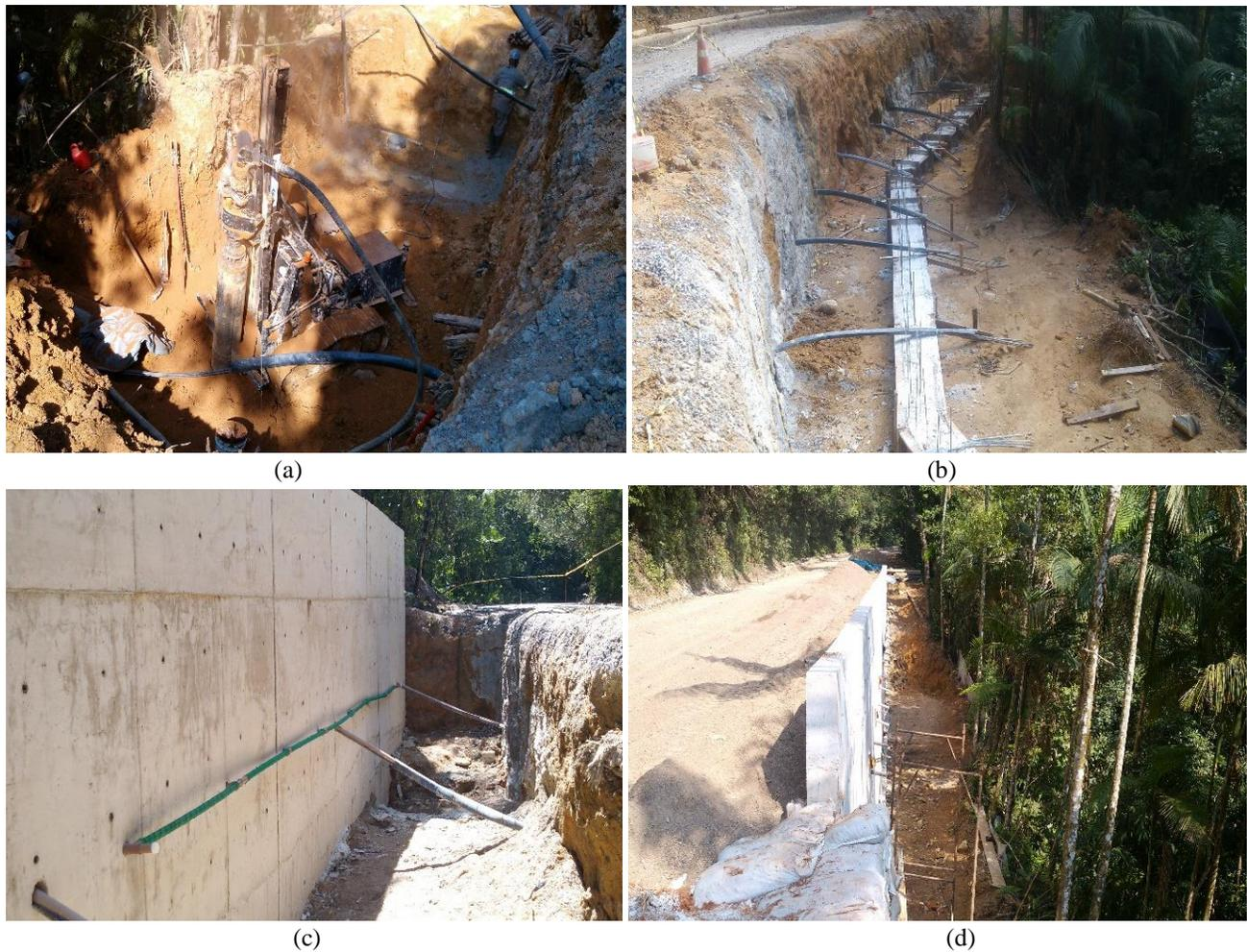
Figure 5. (a) execution of the root pile, (b) general view of the ties incorporated into the curtain, (c) detail of the drainage system, (d) geometry of the track reconstituted with sand.
